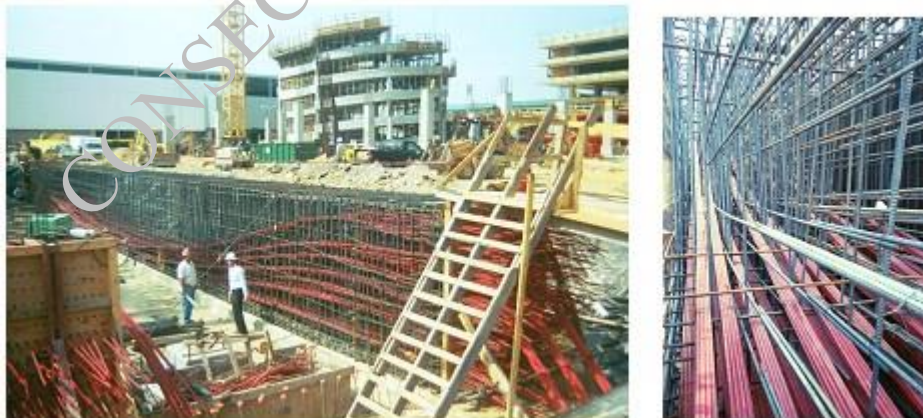
Figure 5. Transfer Girders that bridge over ITT Tunnel at Bush IAH Airport (Courtesy – Suncoast Post-tension Ltd)
