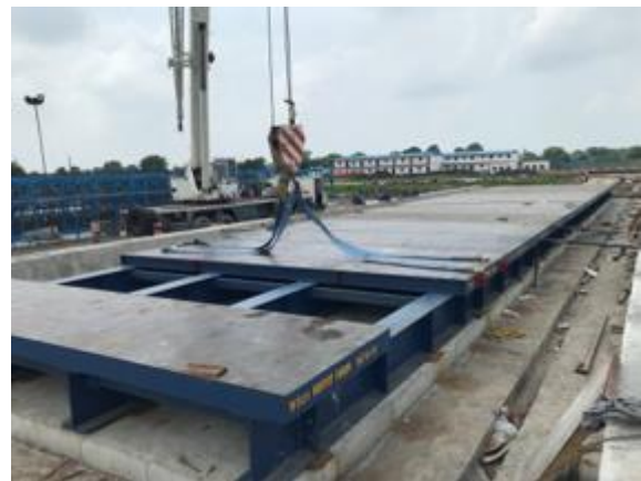
Figure D. Laying of Skin Plates of Outer Shuttering Formwork
