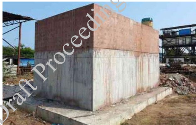
Figure 2. Completed heavy density slab
