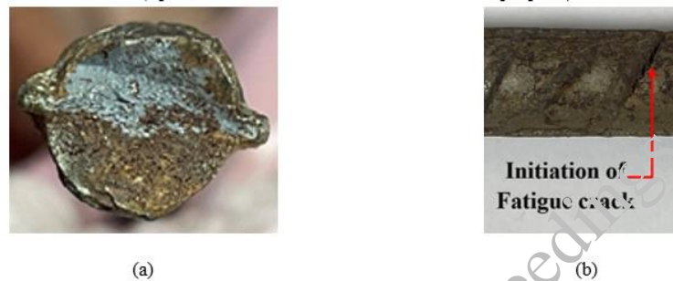
Figure 3. Photograph showing (a) Fracture surface (b) Crack initiation in rebar under fatigue loading in corroded specimens
