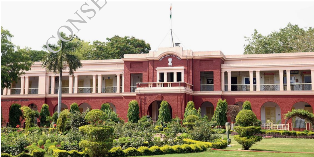
Figure 1. Front View of Heritage Building of IIT (ISM) Dhanbad
